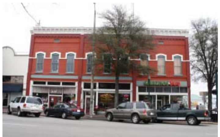
The Loyd Building is an Italianate Style retail structure that is located within the LaGrange Commercial Historic District. Photo by Joy Melton
