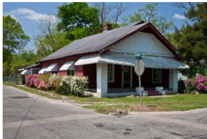
The exterior of the Georgia B. Williams Nursing Home looks very much like the neighboring houses. The front door opened into Ms. Borders' living quarters, while maternity patients and their families used the side door.
