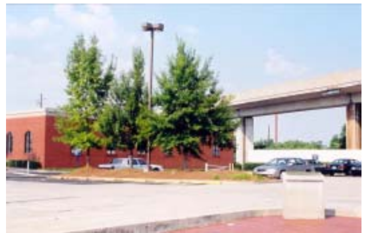
This current view shows the historical plaque erected in 1937 at the site of the old White Hall tavern and post office in West End. A Wachovia Bank branch and the MARTA rail lines have replaced the First National Bank branch and the old rail terminals. Photo by Jeanne Cyriaque
