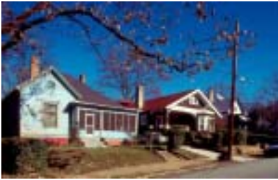
These circa 1900-1930 Craftsman-style bungalows are the most prevalent house type in the West End Historic District. Photo by James R. Lockhart
