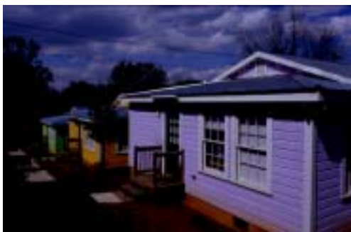
In 1996, the current owner rehabilitated these homes and qualified for the tax incentives program of the National Park Service. Photo by James R. Lockhart
