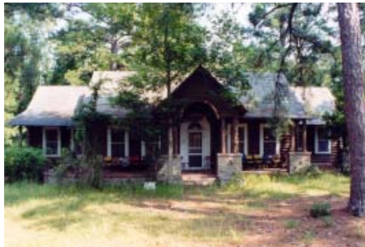
The Camilla-Zach Country Life Center was built by Benjamin F. Hubert in honor of his parents. The log cabin center is one of the buildings in the Camilla-Zach Community Center historic district, listed in the National Register of Historic Places on December 2, 1974. Photo by Jeanne Cyriaque
