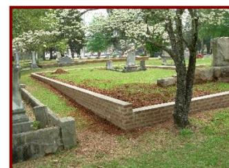
broken tombstones, sunken ledgers, collapsed brick-over tombs, and badly stained monuments. Additionally, tree roots and limbs, soil erosion, acid rain, and lichen growth had also taken their toll on the cemetery. The grant project included coping (see photos above), walkway, ledger and tomb repair, as well as tree removal.
