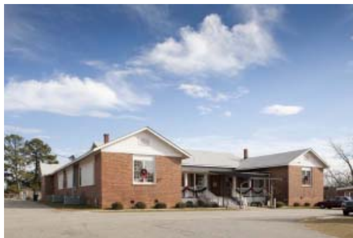
Vienna High and Industrial School is an excellent example of a Rosenwald Community School Plan building that was constructed to accommodate six teachers in three classrooms on each side, an auditorium, and a principal's office. Photo by James R. Lockhart
