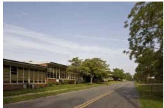
This portion of the former Douglass Junior High School was constructed in the 1950s. Photo by James R. Lockhart
