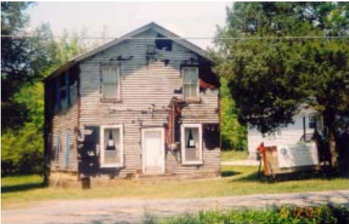
*The preservation plan revealed several structural deficiencies and safety issues. The red asphalt siding was removed and revealed the original wood siding.*
