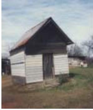
*The smokehouse on the Morgan farm features a raised-seam, metal roof, and a log foundation. It was built circa 1890 and used until 1993.*
