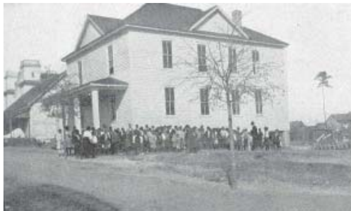
The Vidalia High and Industrial School was a two-story school built according to plans developed by architects at Tuskegee Institute. These plans were used until the Julius Rosenwald Fund developed Community School Plans in 1920. Source: Georgia Dept. of Education 1918 Annual Report
