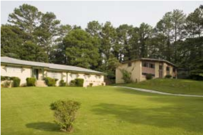
The Ranch house on the left uses metal shutters for ornamentation. The house on the right is a Split-Foyer. Its distinctive characteristics are an entrance at grade level with the main living area on the upper level while the lower level provides ample space for a recreation area. Photo by James R. Lockhart
