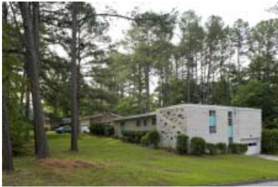
This Modern Split-Level house incorporates International Style elements with a flat roof and stones interspersed with the brick for ornamentation. Photo by James R. Lockhart
