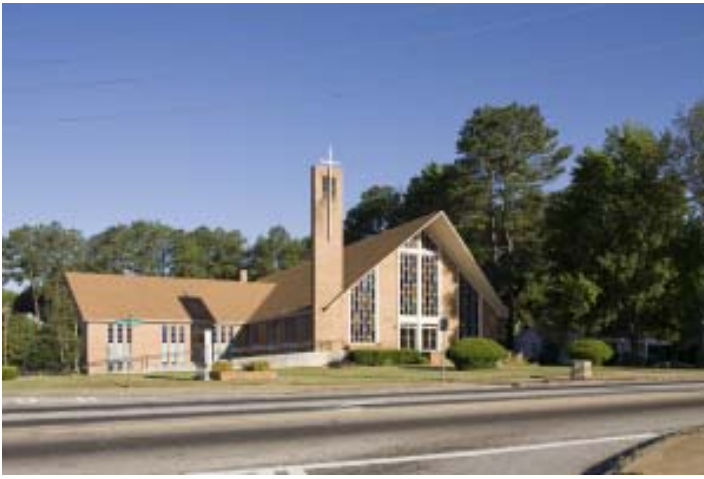
The First Missionary Baptist Church moved to Collier Heights in the 1960s. This church is a Contemporary-style A-Frame with an elongated T-shaped plan. Photo by James R. Lockhart
