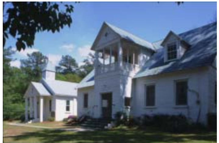
Evergreen Congregational Church and School were listed in the National Register of Historic Places on October 31, 2002. These landmark buildings are excellent examples of an early 20th century church and school complex in a rural African American community. Photo by James R. Lockhart
