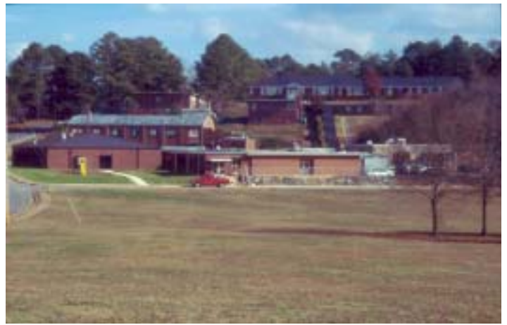
The Main High School campus includes the 1934 Colonial Revival building at the top of a hill. International Style buildings were added as enrollment grew to over 1,200 students.
