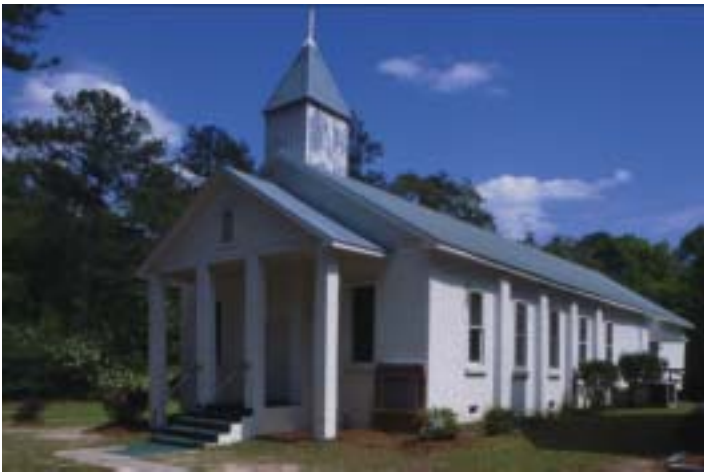
Evergreen Congregational Church was built by church members in 1928. Architectural features include a pyramidal-roofed cupola and a gable-roof portico supported by four posts. Photo by James R. Lockhart
